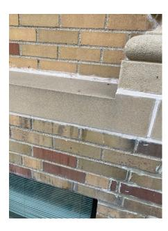
Remove, grind to 1" depth, point back, rake joint, install backer rod, re-caulk water table head joints and top & bottom bed joints
