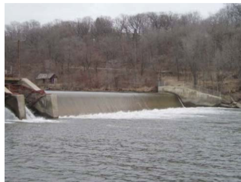
View of the Ogee crest spillway
