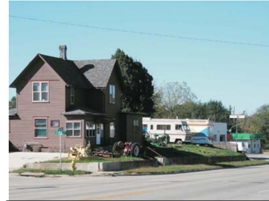
Before: 19th Street & 5th Ave existing residential/commercial development
