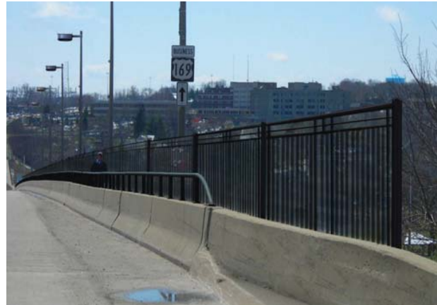
Bridge Enhanced with New Ornamental Railing
