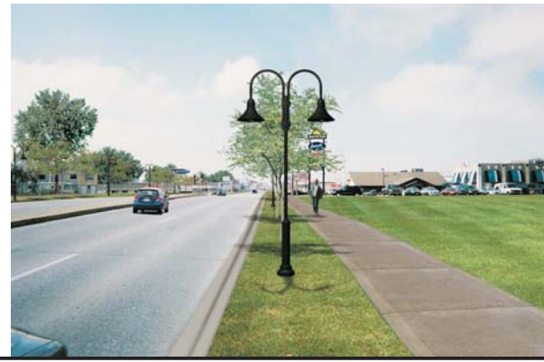
After: 5TH Ave/Hwy 20 - Buried overhead utilities & new streetscape
