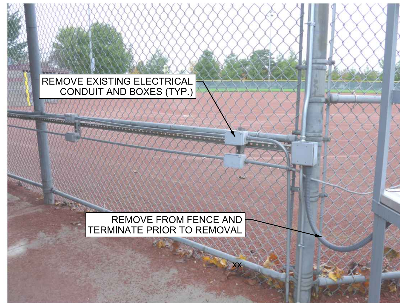
EXISTING ELECTRICAL/COMMUNICATION SYSTEM - PRESS AREA
